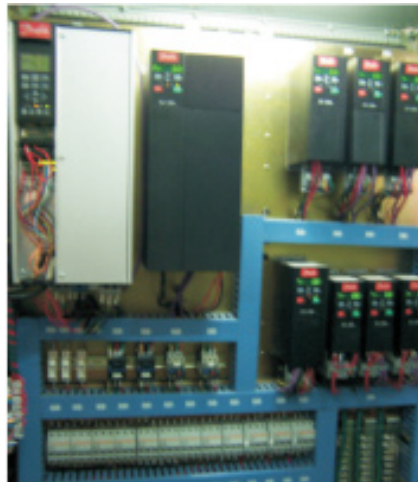
Fig. 2 Wiring of the Frequency Converter
